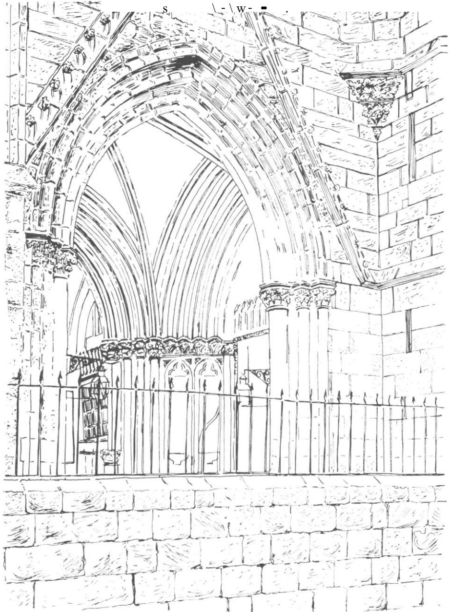
Fig. 66 Encorbelment on southern tower.
