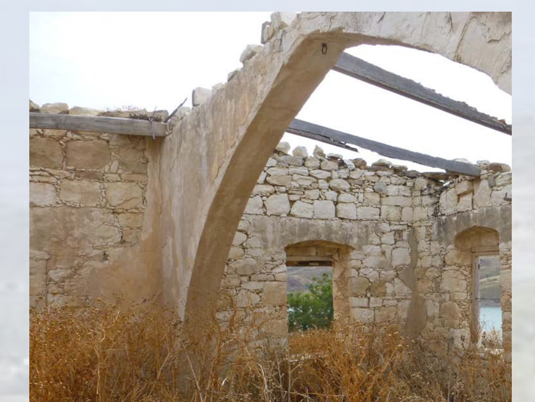
Building 1 rubble stone masonry, interior arch, and roof timbers.
