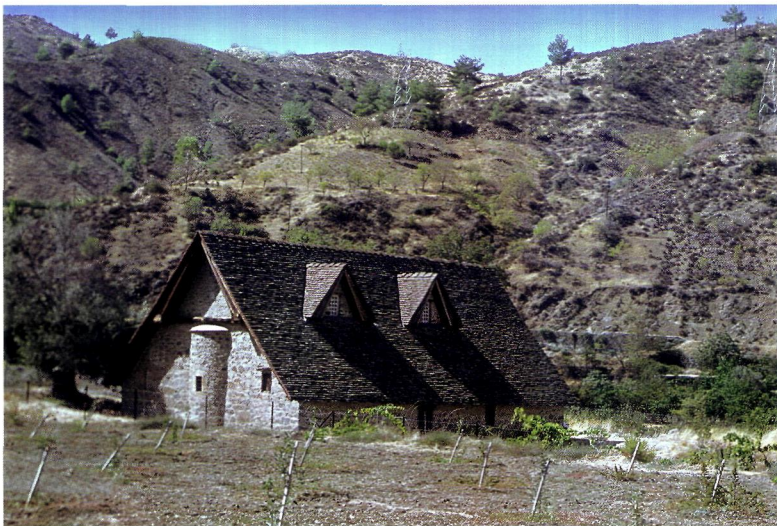
45. The church of Panagia Podithou, 1502, Galata. (The ventilators in the roof are modern additions to this type of architecture in the island, and they will be removed as soon as electricity is installed in the church).
